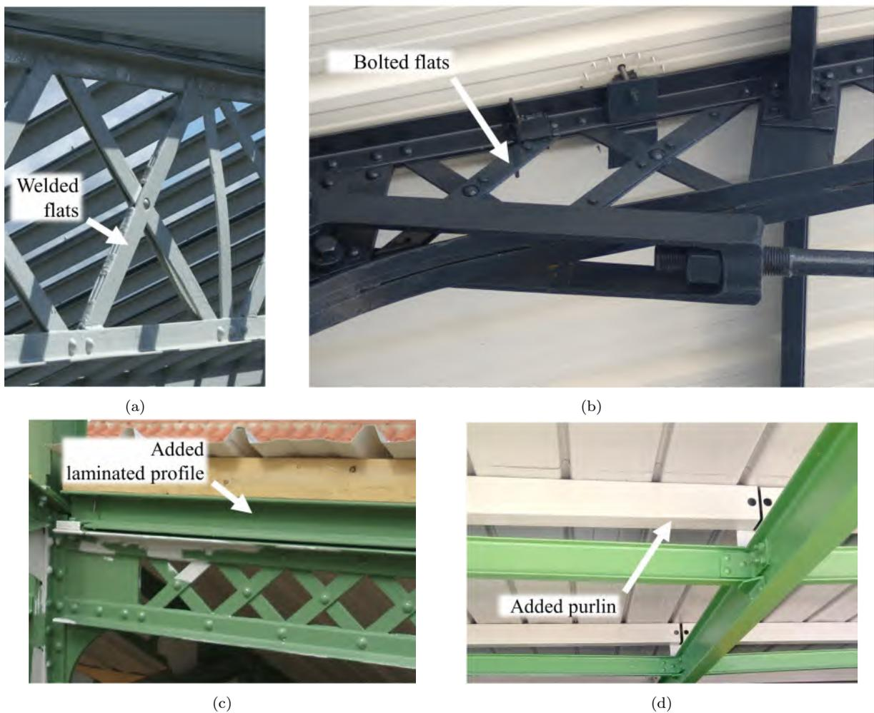
Figure 2.15 – Interventions increasing the cross-section of existing elements or replacing them (Pictures from SNCF-AREP). (a) Welded flats, Gare de Montauban, Montauban, France; (b) Bolted flats on existing diagonals, Gare d’Hendaye, Hendaye, France; (c) Added rolled steel section on top of existing lattice purlin, Gare de Cerbère, Cerbère, France; (d) Added tubular purlins effectively replacing the existing ones, Gare de Béziers, Béziers, France.
