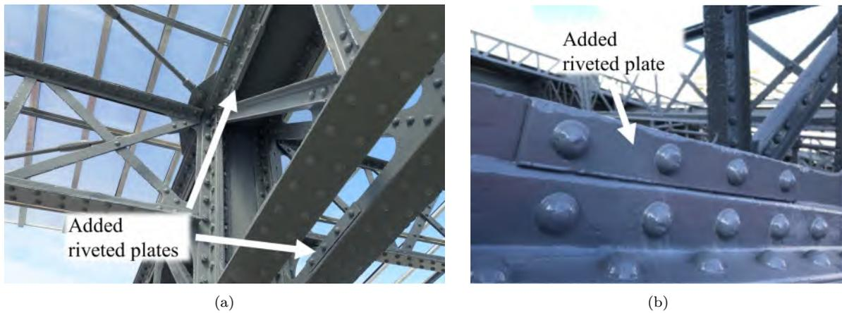
Figure 2.12 – Local repairs of roof truss chords with added riveted plates in the train shed of Troyes renovated in 2021, Troyes, France (Pictures from SNCF).
