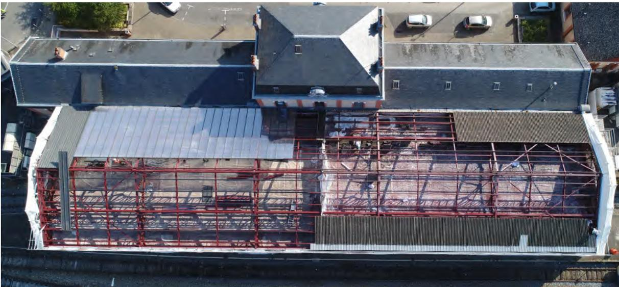
Figure 2.1 – Example of complete replacement of the roofing: aerial view of the restoration of the shed of the Gare de Tulle in 2019, Tulle, France (Picture from SNCF). Right side: old fibre cement panels. Left side: new steel decks and polycarbonate panels.
