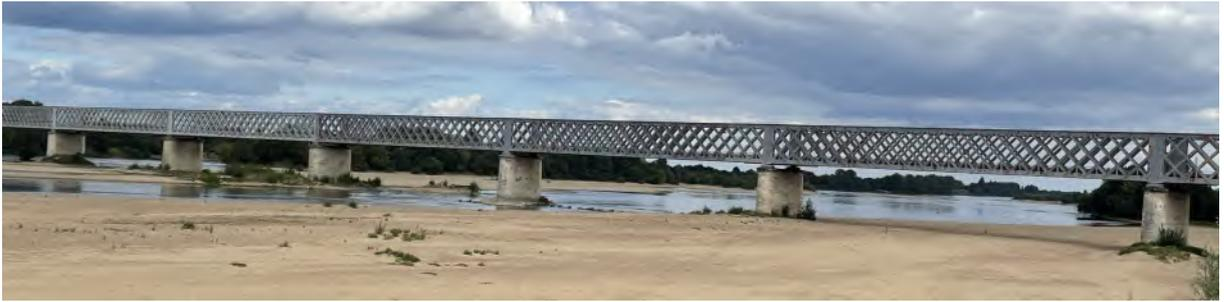
Figure 1.10 – Lattice bridge across the Loire - Pont de Varennes-Montsaureau, built in 1917 (Picture by H. Franz).
