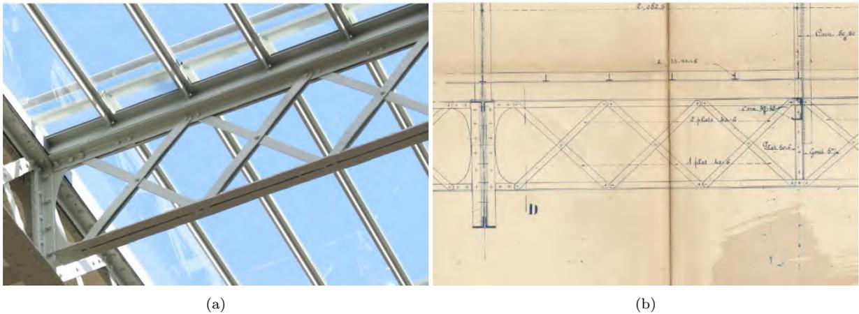
Figure 1.13 – Repeated construction details in train sheds built by same contractor Daydé et Pillé (Picture from SNCF-AREP, archive plan from SNCF archives): (a) Gare de Montaubau, detail of a lattice purlin, Montauban, France; (b) Gare de Bédarieux, detail of a lattice purlin from an archive plan, Bédarieux, France.
