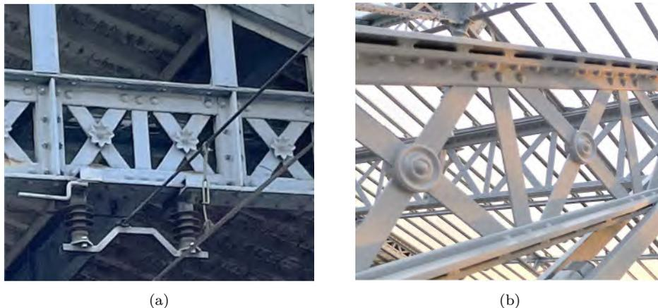
Figure 1.11 – Examples of ornamental additions on lattice IXI-type beams: (a) Gare de Blois, Blois, France (Picture by H. Franz); (b) Gare d’Austerlitz, Paris, France (Picture from SNCF-AREP).
