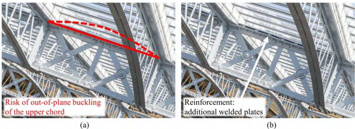
Figure 2 – Example of strengthening measure carried out on a riveted lattice girder because of the predicted buckling risk: the rafters of the train shed of Gare d'Austerlitz, Paris, France. (a) Predicted buckling shape for the upper chord of the lattice rafter; (b) Reinforcement implemented in 2015 (Pictures from SNCF-AREP by M. L. Vigneau).
