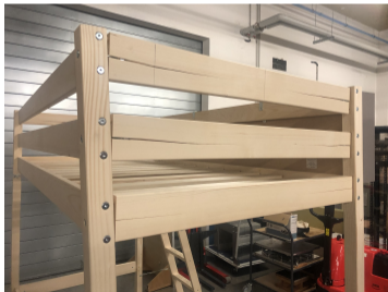
(a) Crossbeams cracking at bunk beds connections
