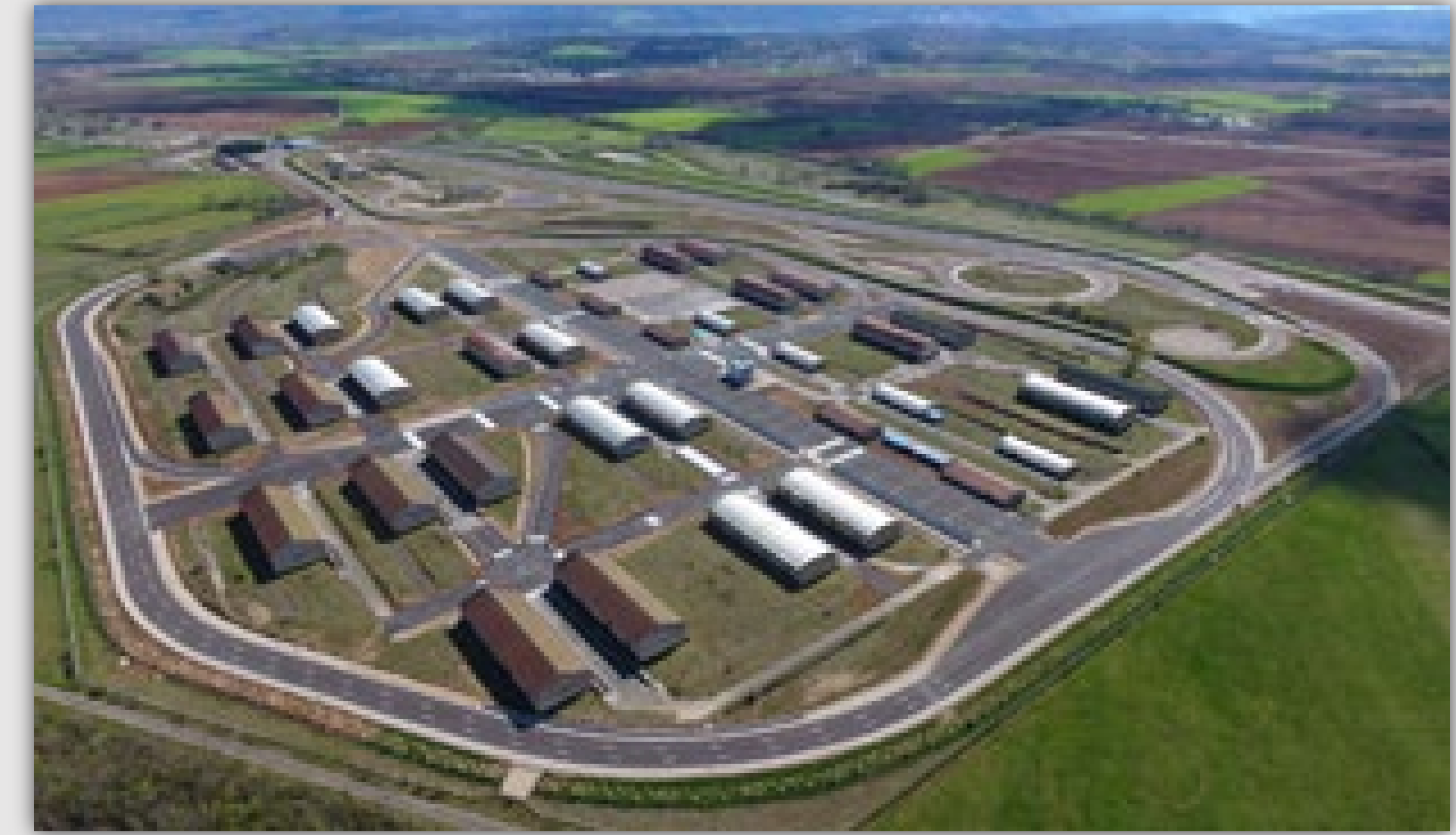
Figure 3 : Aerial view of Transpolis site
