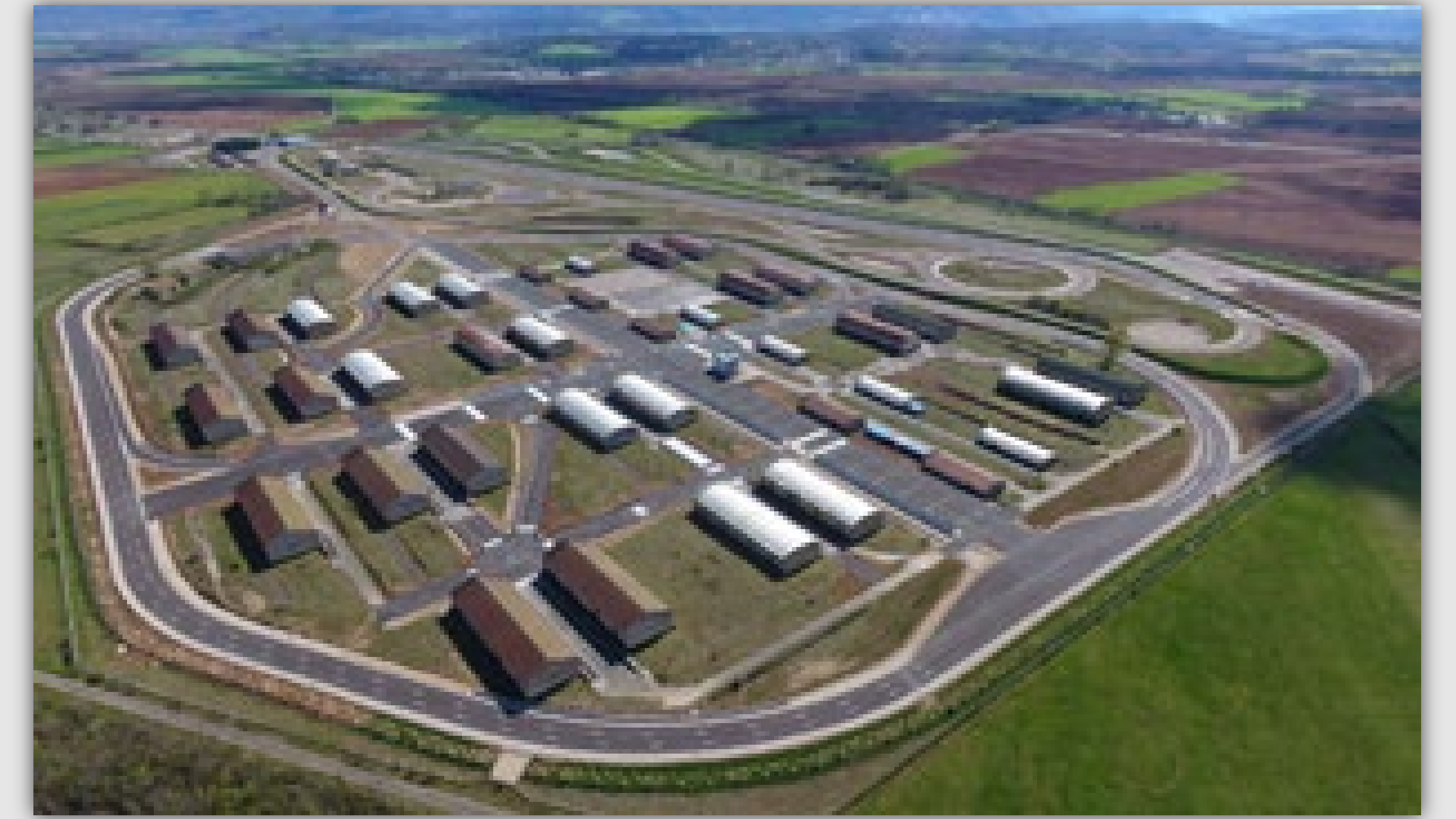
Figure 3 : Aerial view of Transpolis site
