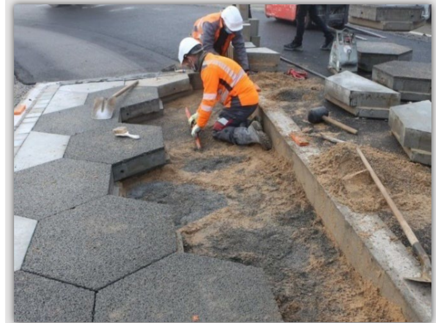
Figure 4 : Installation of RUP test structure at Gustave Eiffel University
