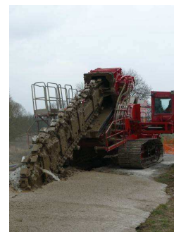
Figure 1. Dry method for soil mixing reinforcement (a) pre-trenched zone and cement powder, (b) production and (c) end of mixing.
