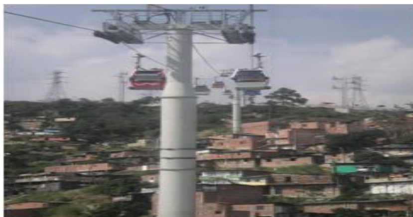
Figure 1: Mono-cable ropeway in Zaragoza-Spain
