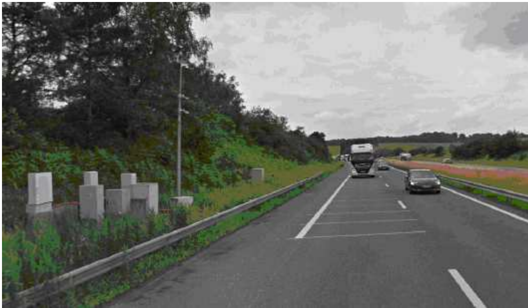
Figure 4: Test site of Saint-Avoid (A4)
