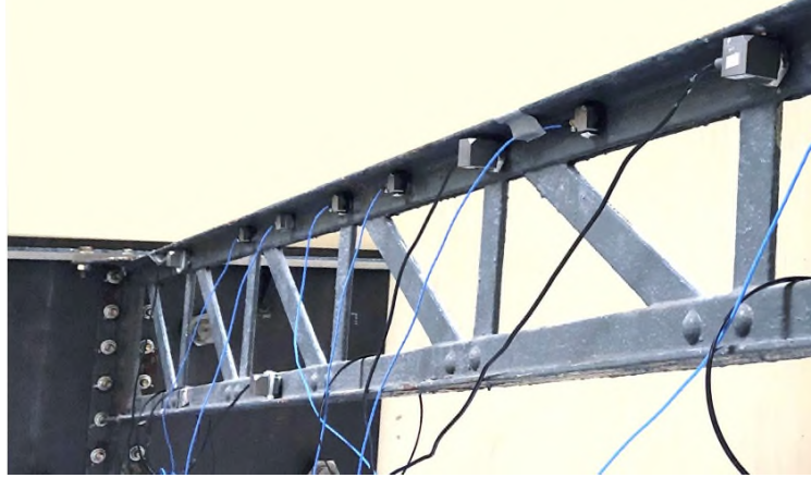
Figure 5: View of the instrumented girder in the laboratory.
