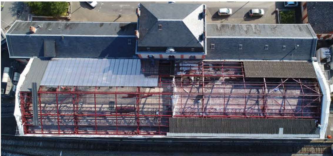
Figure 15 : Example of complete replacement of the roofing: aerial view of the restoration of the shed of the Gare de Tulle in 2019, Tulle, France (Picture from SNCF). Right side: old fibre cement panels. Left side: new steel decks and polycarbonate panels.
