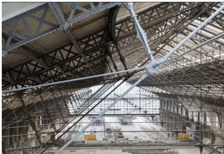
Figure 2: Gare de Paris-Austerlitz, built in 1869, under restoration in 2016, Paris, France (Picture from SNCF-AREP by M. Lee-Vigneau).
