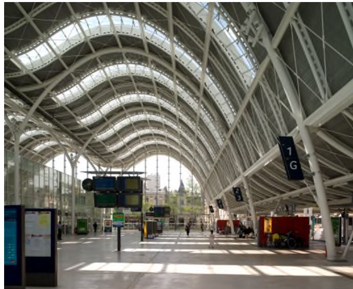
Figure 28: Gare d'Orléans, built in 2009, Orléans, France (Picture from SNCF-AREP by D. Boy de la Tour).
