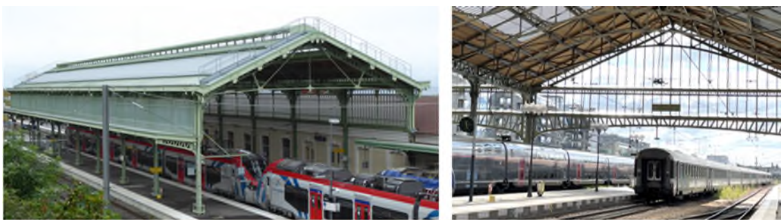
Figure 14 : (a) Skylight along the ridge (Gare d'Evian, Evian, France) (Picture from SNCF). (b) Glazed gable (Gare de Tours, Tours, France) (Picture from H. Franz).
