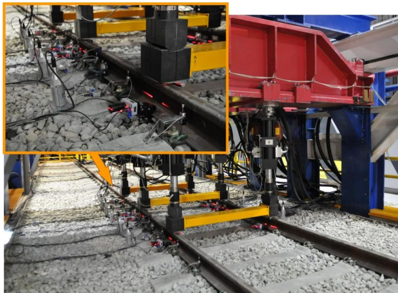
Figure 84 Surface instrumentation installed in one test
