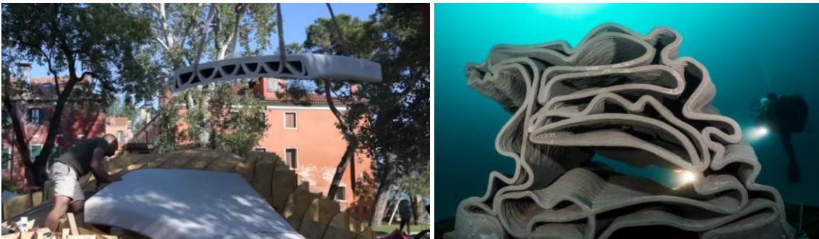
Figure 4-54 Printed and unreinforced concrete bridge on left (ETH Zurich, 2021). Artificial reef on right (XtreeE, 2017).
