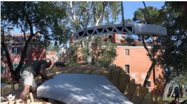
Figure 4-54 Printed and unreinforced concrete bridge on left (ETH Zurich, 2021). Artificial reef on right (XtreeE, 2017).
