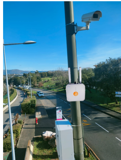
Fig. 1. The information system consists in a camera attached to a public lighting pole, watching road-side parking slots in the City of Biot, France. The camera is connected to a computer in a box and a road-side unit (added on the image).
