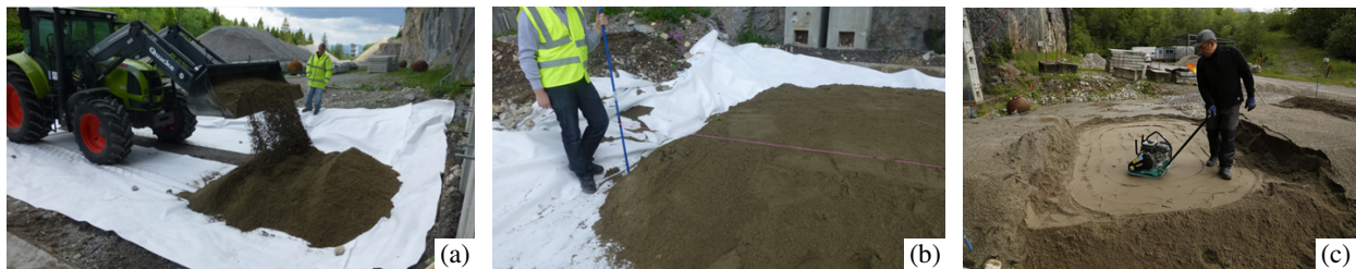
Fig. 4. (a) Soil dumping on geotextile using a backhoe; (b) Leveling of the soil sub-layers and (c) soil compaction using a vibrating plate compactor.
