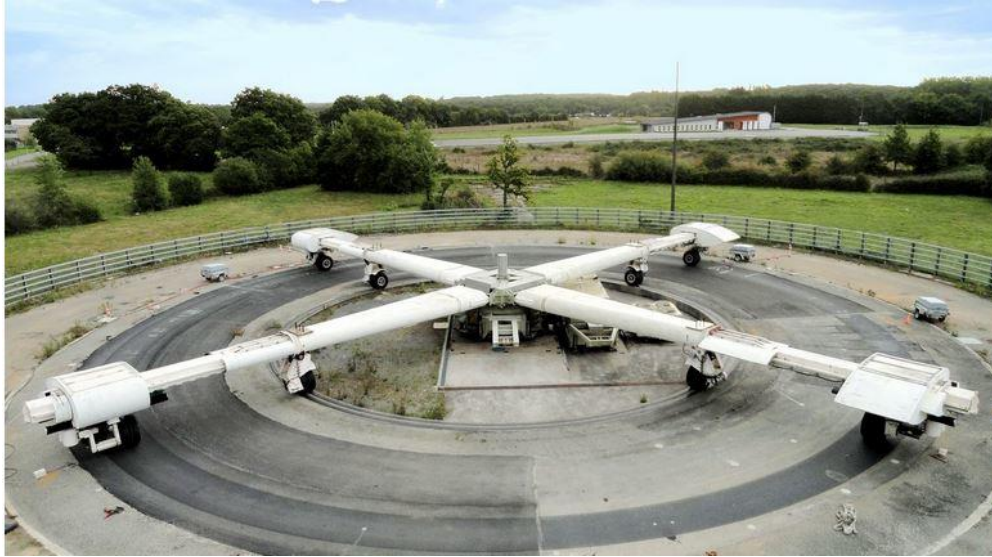
Figure 1: The pavement fatigue carousel at university Gustave Eiffel (Nantes campus)
