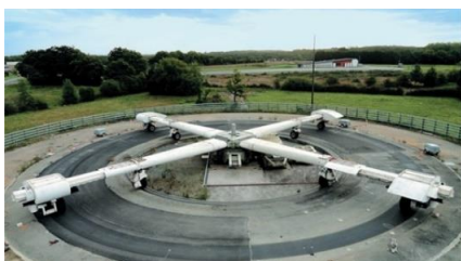
Fig. 4. Image of fatigue carousel platform in Gustave Eiffel University (Nantes/France)
