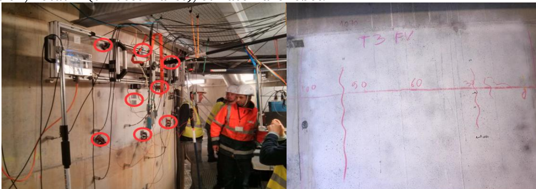
Figure 7. Instrumentation for acoustic emission, diffuse waves (Locadiff) and surface wave robot set up to monitor to follow the cracks: Inspected zone with in red vertical cracks.
