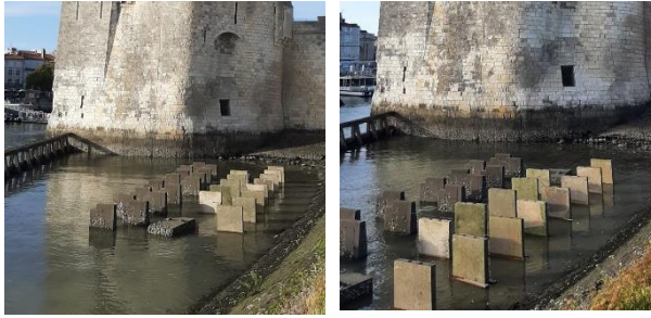
Fig. 9. During the tide's descent, the bottom of the walls remains a longer time immersed.
