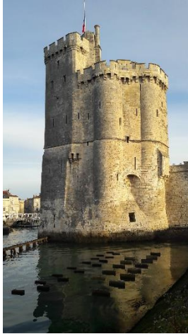
Fig. 10. At high tide of low coefficient, the top of the walls remains in the open air.
