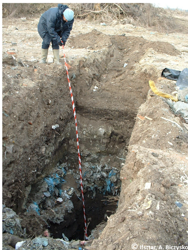
Figure 7. Picture of the excavations in the “Prairie de Mauves” waste deposit.
